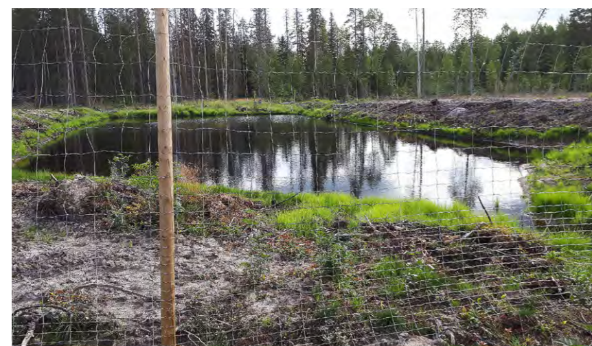
Photo and illustration of a sedimentation pond with a distribution ditch before an overland flow area. Sedimentation ponds are built in larger ditch networks. Photo: Sixten Karlsson. Illustration: Bo Persson
