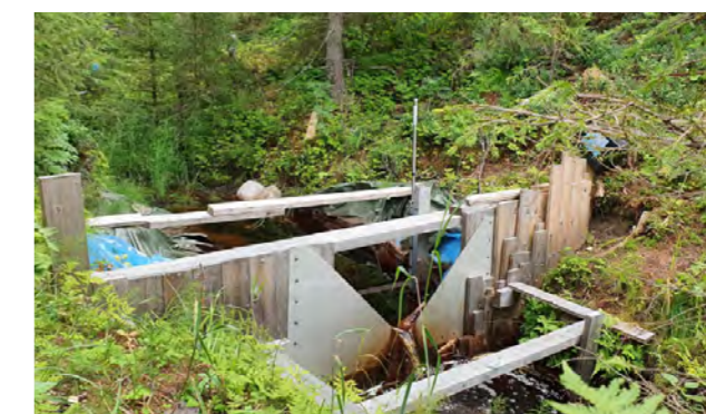
V-notch flow measuring stations are located by the outlets of all the catchments to monitor effects on water quality and quantity. Photo Tobias Eriksson
