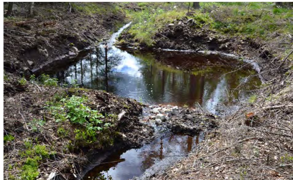
Example of a sedimentation pit. The inlet and outlet ditch are laterally offset from each other to slow down the water velocity and extend the retention time. The outlet ditch is also shallower than the inlet ditch. Photo: Daniel Palm
